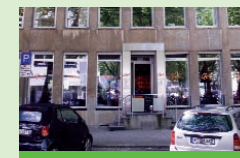
Church: Restaurant und Depot III. Hagen 39
